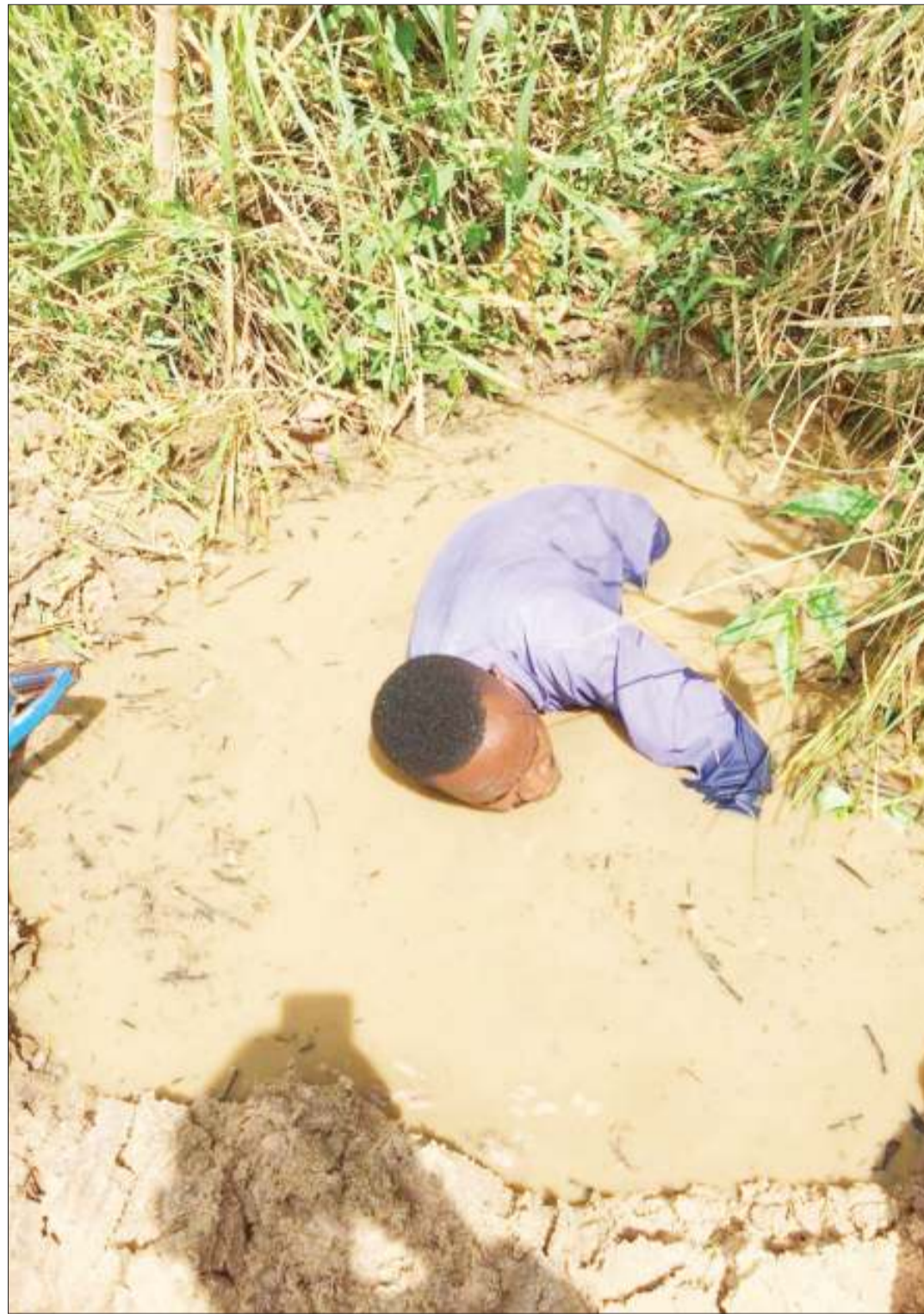
Commitment: Dar es Salaam Water and Sewage Authority employee at Tegeta in the outskirts of Dar es Salaam seals water pump leakage at Bunju B in Kinondoni on Tuesday. Dawasa commits to reduce water leakages by 35 per cent by next year. Photo: Guardian Correspondent
