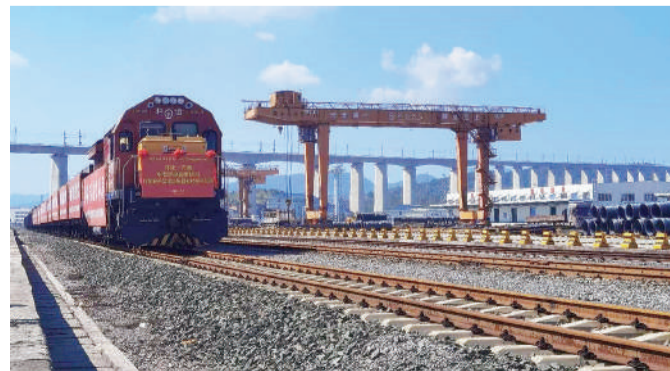
A fully loaded train departs from Huaihua, central China's Hunan province, heading towards Vientiane, Laos along the China-Laos Railway, Oct. 30, 2023. Photo: Tian Min/People's Daily Online
