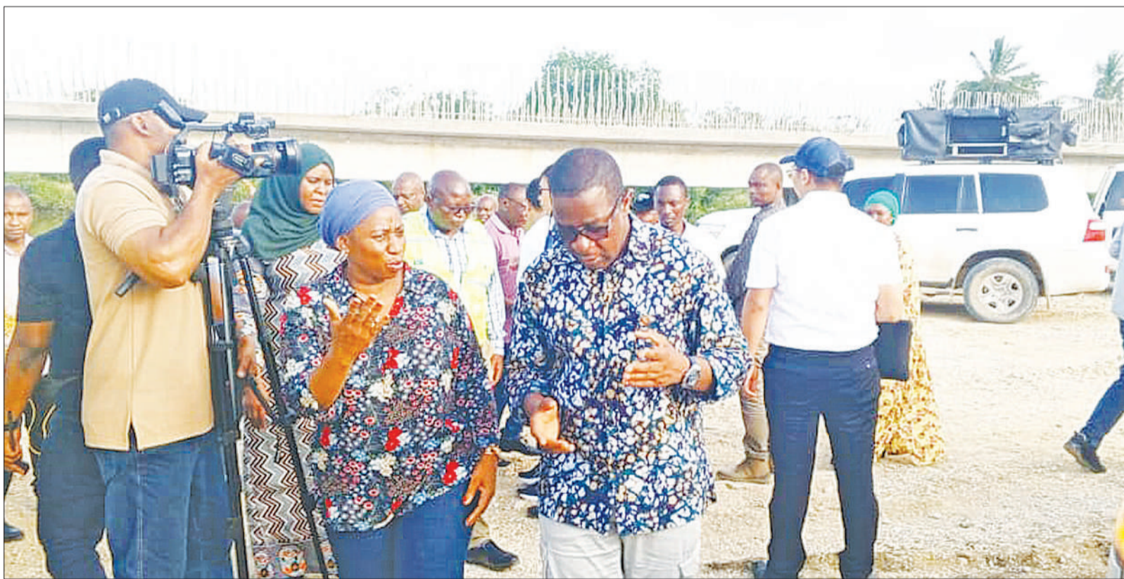
Tanga Urban MP Umyy Mwalimu (L), speaks with Works minister Abdallah Ulega, while on a visit to inspect the construction of the Tanga-Pangani road. Photo: Correspondent Oscar Assenga
