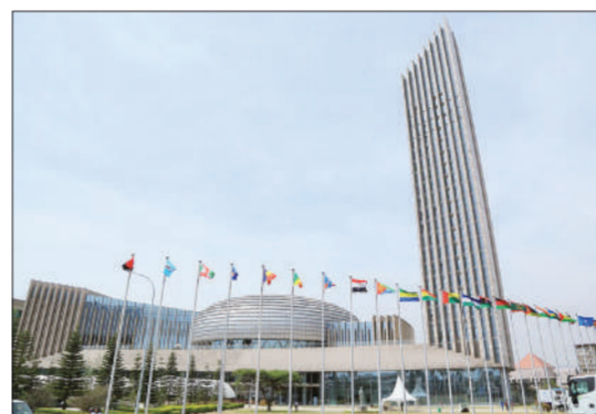
Photo taken on Feb. 3, 2022 shows the buildings of the African Union (AU) headquarters in Addis Ababa, Ethiopia. (Xinhua)
