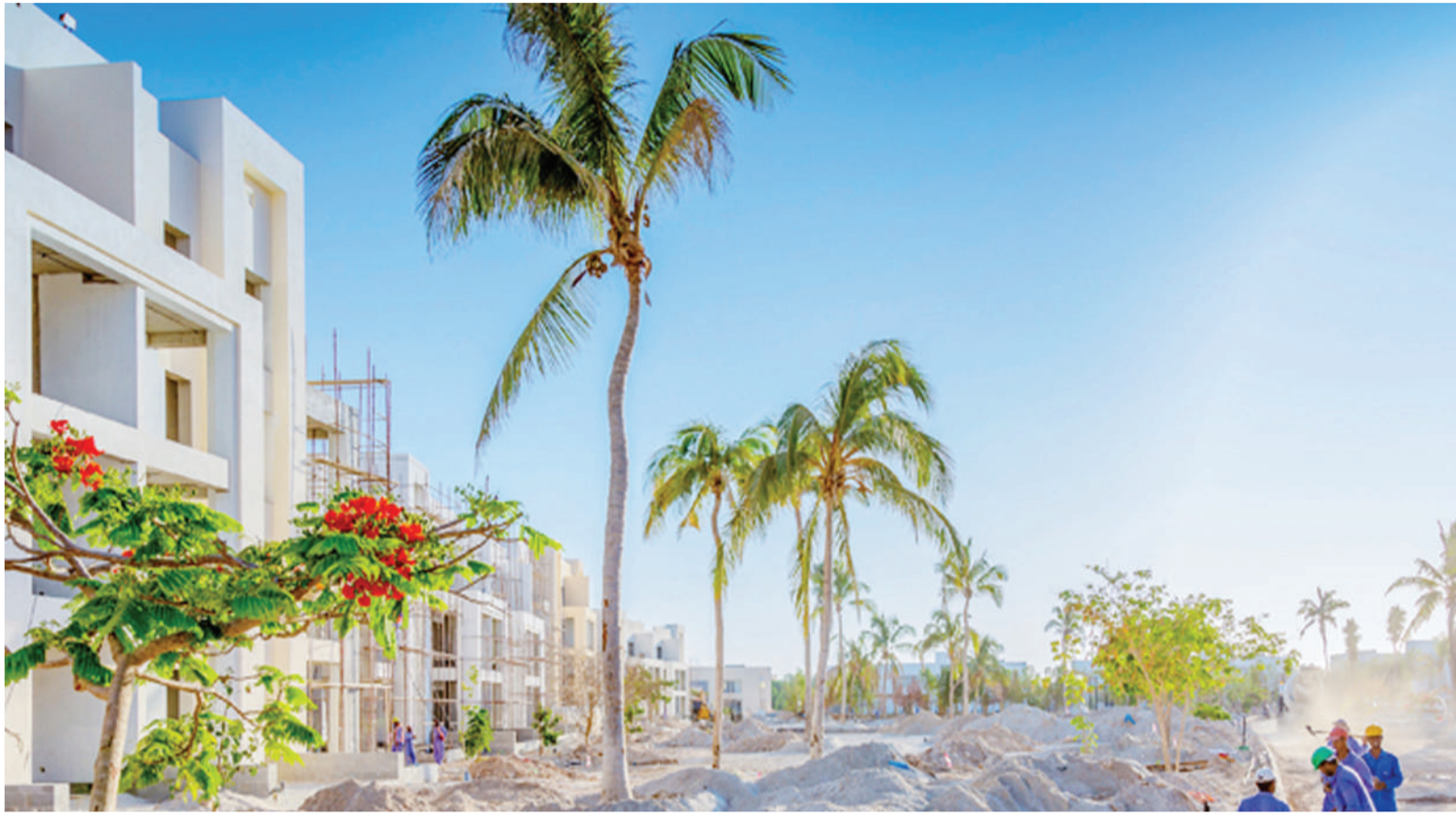
Construction work going on at Muriya's flagship destination in Hawana Salalah.
