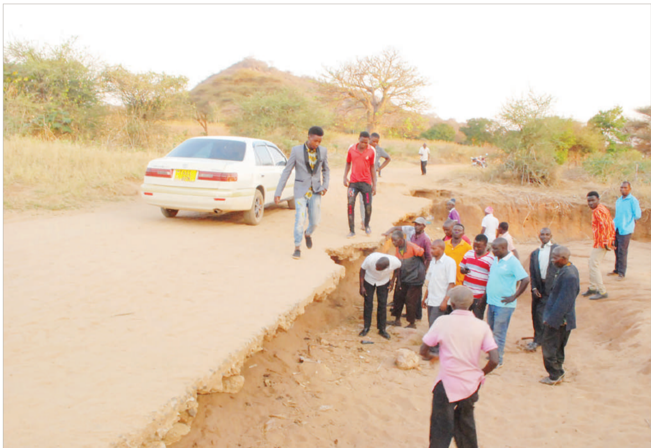
JUST TO BE SURE: Residents of Leganga in Kongwa District, Dodoma Region, pictured yesterday checking a strategic bridge eroded by recent rain. Photo: Correspondent Peter Mkwavila
