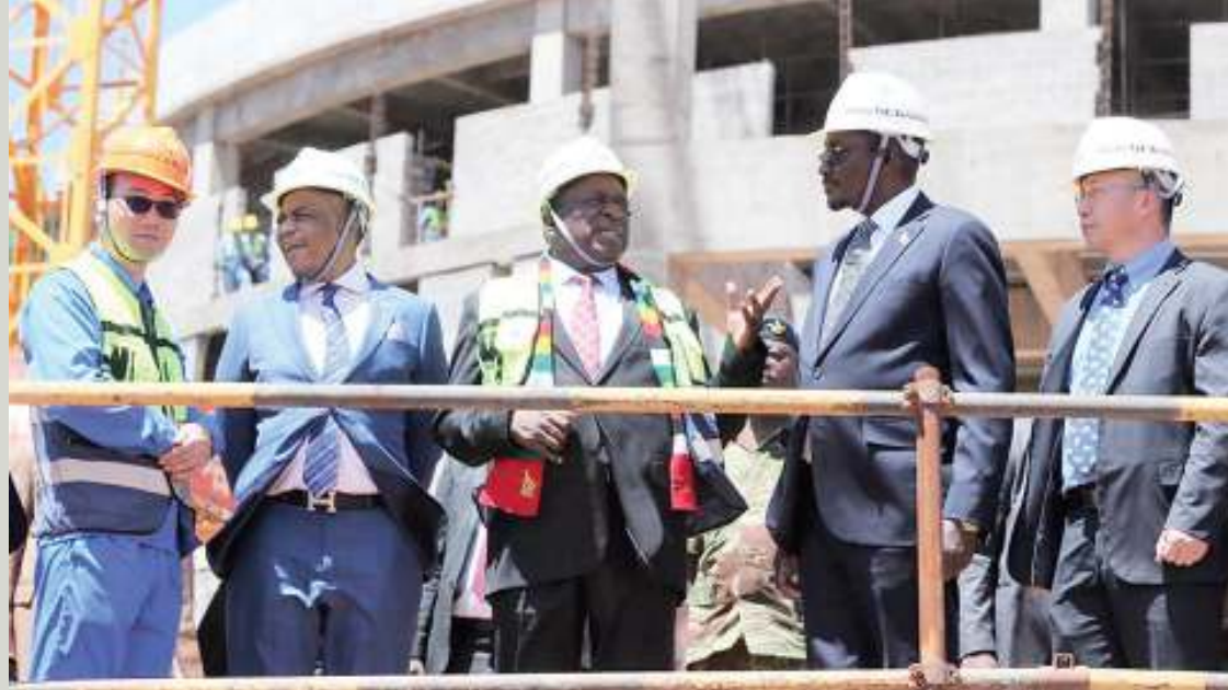
Zimbabwean President Emmerson Mnangagwa (C) inspects the site of the new parliament building in Mount Hampden, about 25 kilometers west of the capital Harare, Zimbabwe, on Wednesday. Zimbabwean President Emmerson Mnangagwa on Wednesday toured the site of the new parliament building that is being constructed by China's Shanghai Construction Group (SCG), and expressed satisfaction with progress made so far. (Xinhua)
