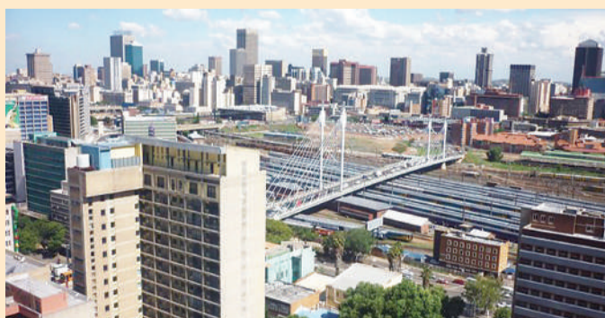
Braamfontein and Johannesburg CBD. Inside a building material shop in Johannesburg.
