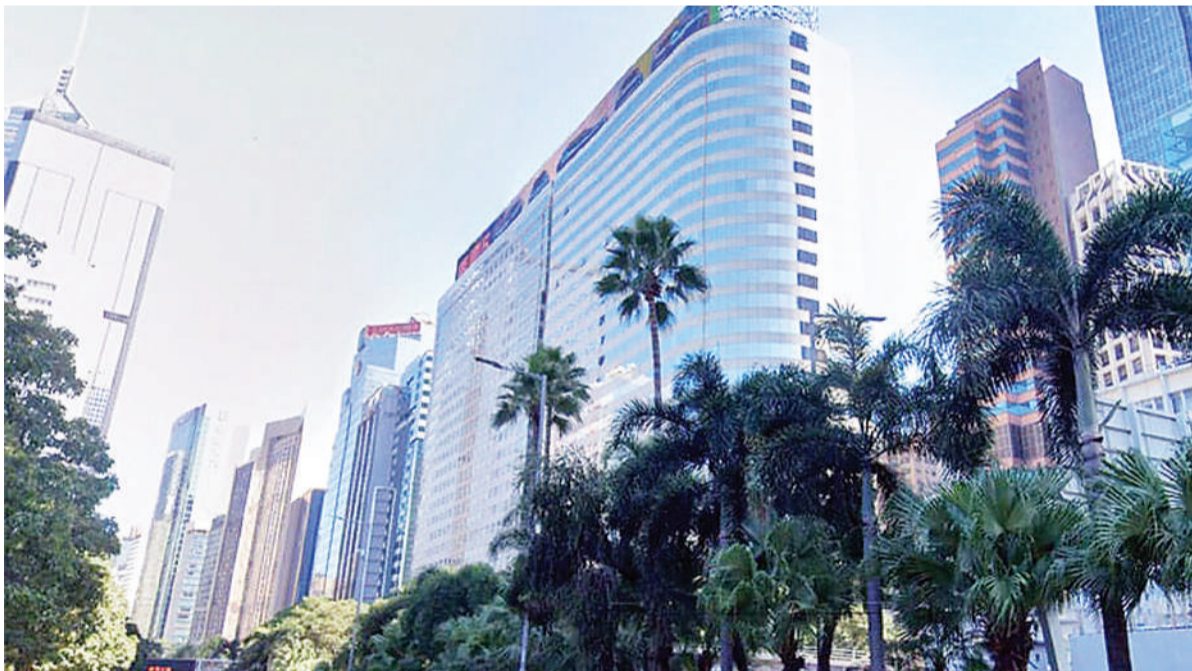
China Evergrande Centre in Wanchai.
