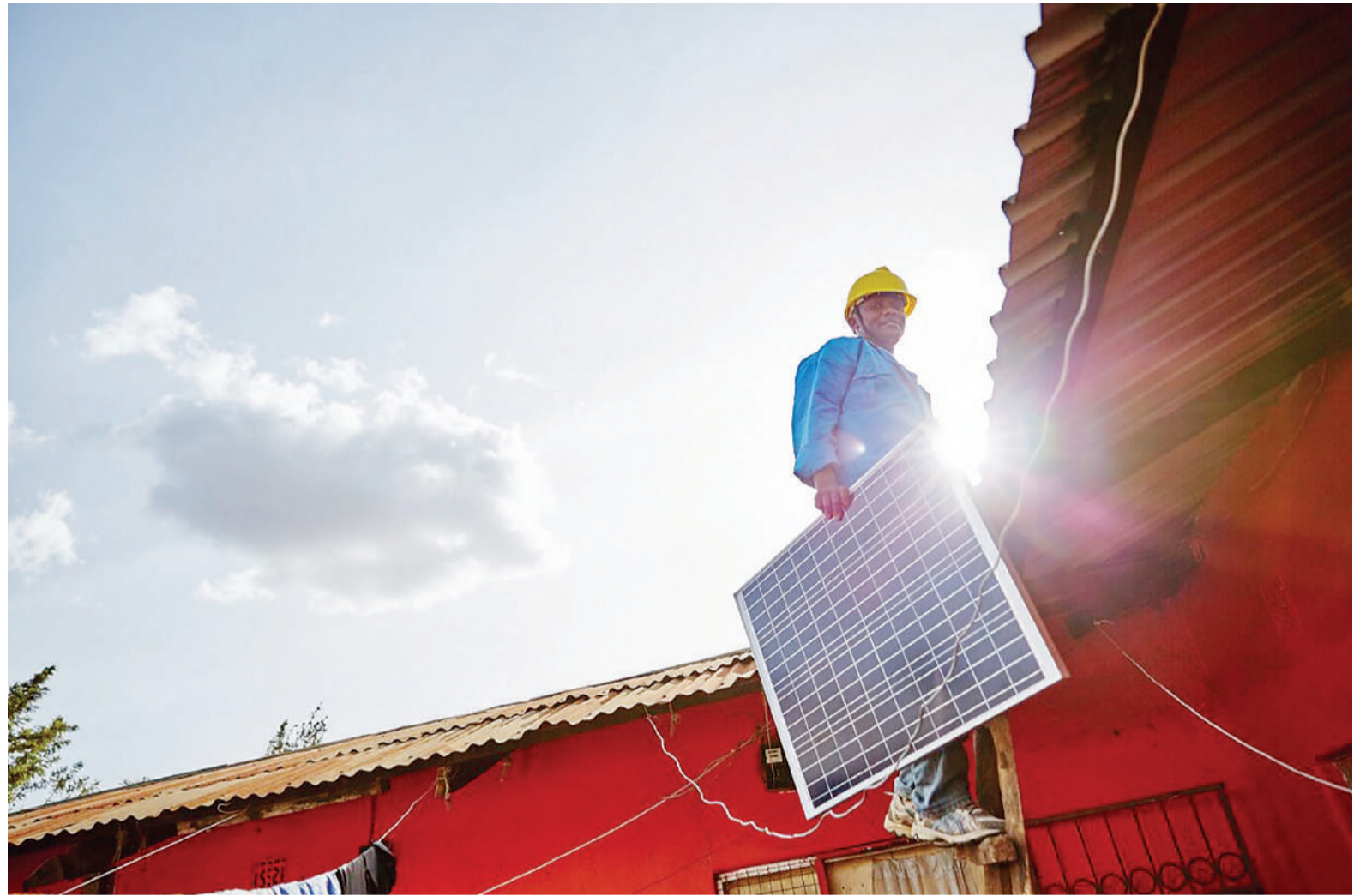
A Zola Electric Limited technician at work.
