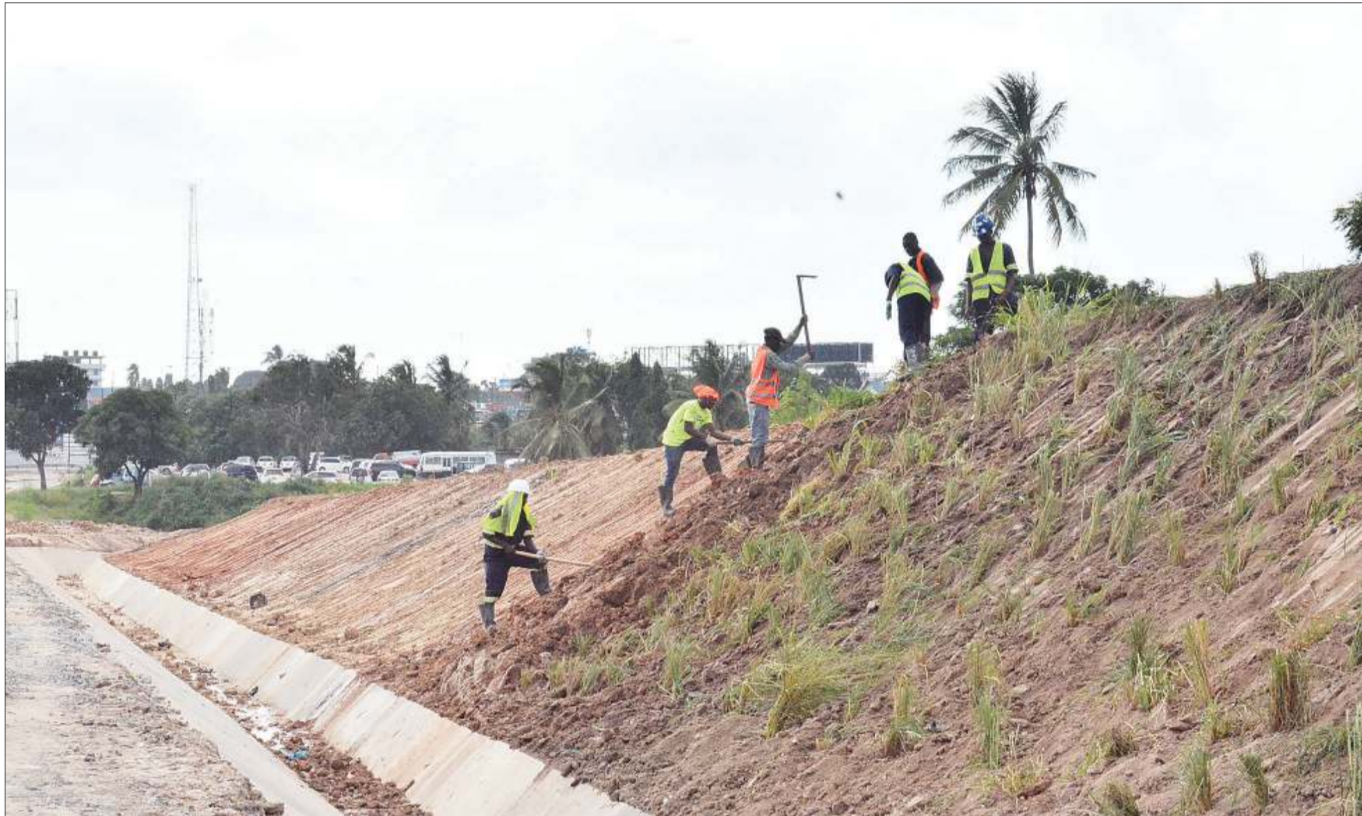
Estim Company workers engaged in the ongoing expansion of the Dar es Salaam-Kibaha stretch of Morogoro Road plant grass at Kimara Mwisho yesterday in an effort to prevent soil erosion and forestall needless damage to the road. Photo: Correspondent Ibrahim Joseph
