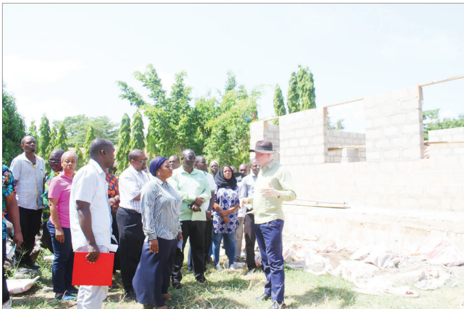
Ernest Kimaya (R), councillor for Chumbageni in Tanga city, briefs Minister of State in the Vice President's Office (Environment), Ummu Mwalimu (C, in headscarf) on the ongoing construction of classrooms at Chumbageni Secondary School. The minister toured the school yesterday. Photo: Correspondent Boniface Gideon
