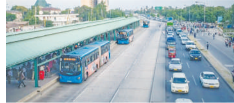
DART TO INSTALL TURNSTILE GATES AT BRT STATIONS PAGE 4
