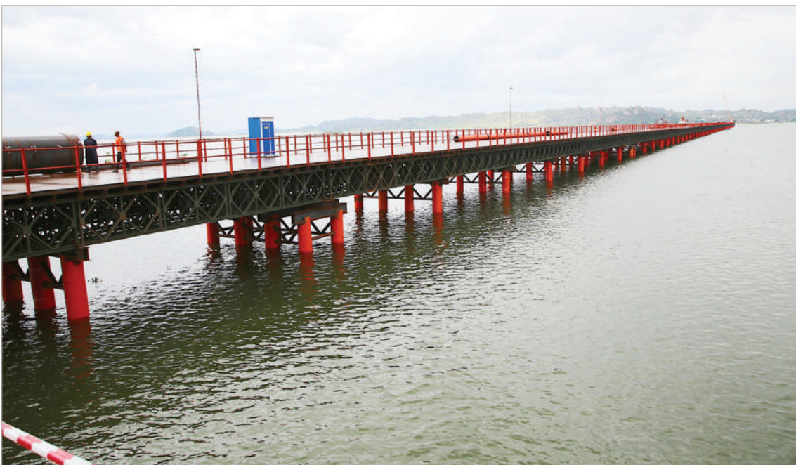
A temporary bridge to haul building materials for the Kigongo-Busisi bridge project that was inspected by Prime Minister Kassim Majaliwa yesterday. Photo: PMO
