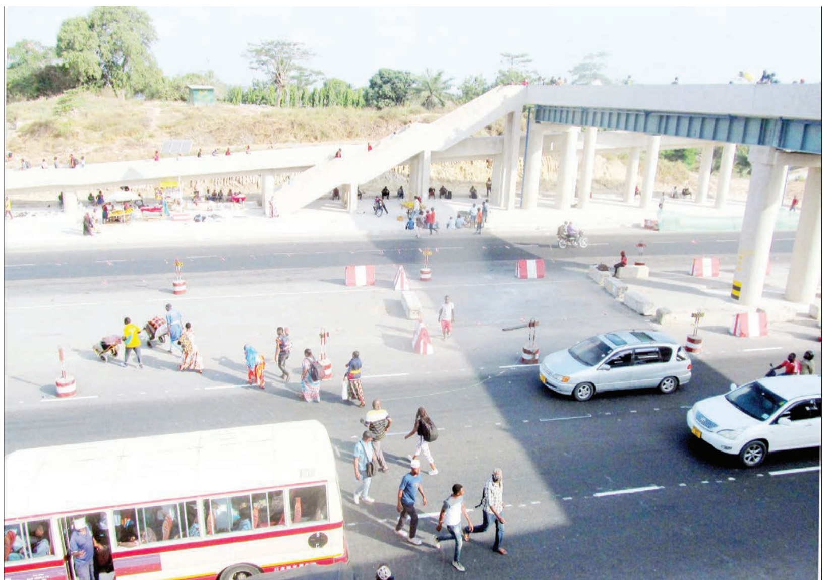
Pedestrians risk endangering their lives by crossing a Mbezi Mwisho section of Morogoro Road in Dar es Salaam yesterday instead of using the overhead bridge (R) meant to forestall needless traffic accidents. Photo: Correspondent Sabato Kasika
