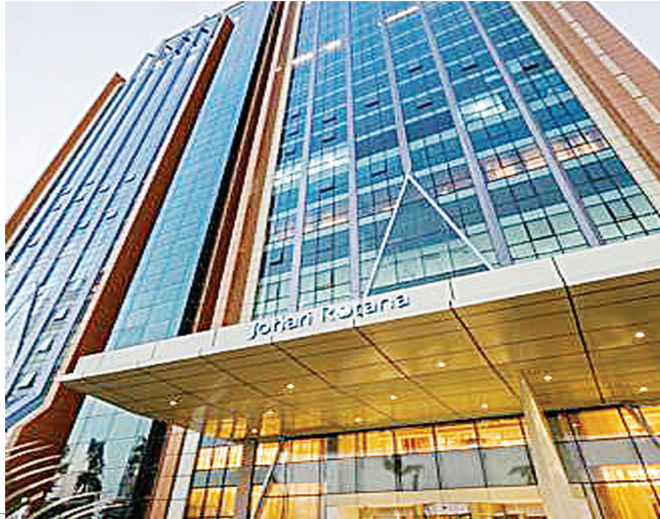
Johari Rotana Hotel in Dar es Salaam.
