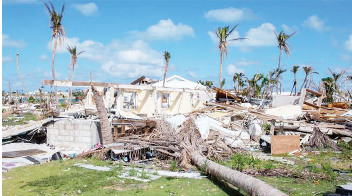
Destruction from hurricane Dorian showing debris and structural damage to buildings and trees in MARSH HARBOR, ABACO ISLAND, THE BAHAMAS. Credit: Shutterstock.
