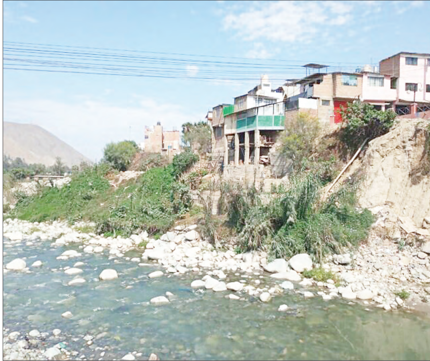
View of the Rimac River as it passes through the municipality of Lurigancho-Chosica, in the Peruvian province of Lima. In this town, many families are still living in housing in areas at high risk, which is exacerbated during the rainy season that begins in December and has intensified due to climate change and the increased recurrence of the El Niño climate phenomenon. CREDIT: Mariela Jara / IPS
