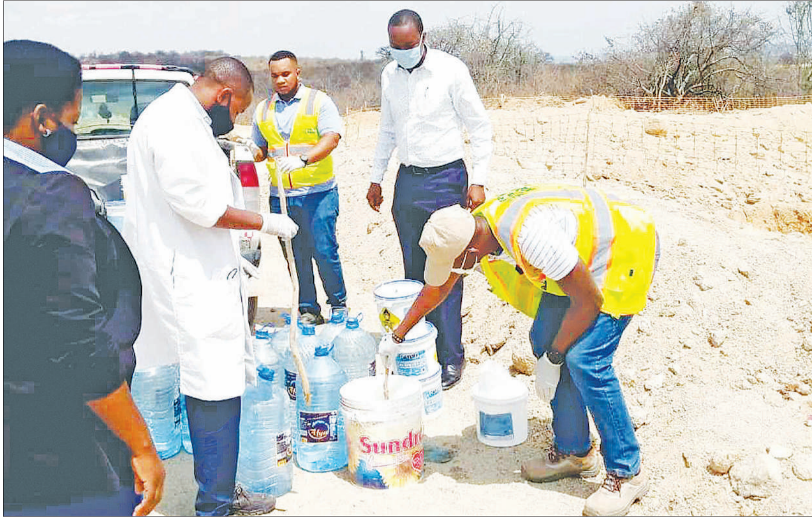
National Environment Management Council (NEMC) officials pictured in Dodoma city earlier this week screening sewage scooped from pits dug by the contractor engaged in the execution of the Standard Gauge Railway project. Photo courtesy of Correspondent Joseph Mwendapole
