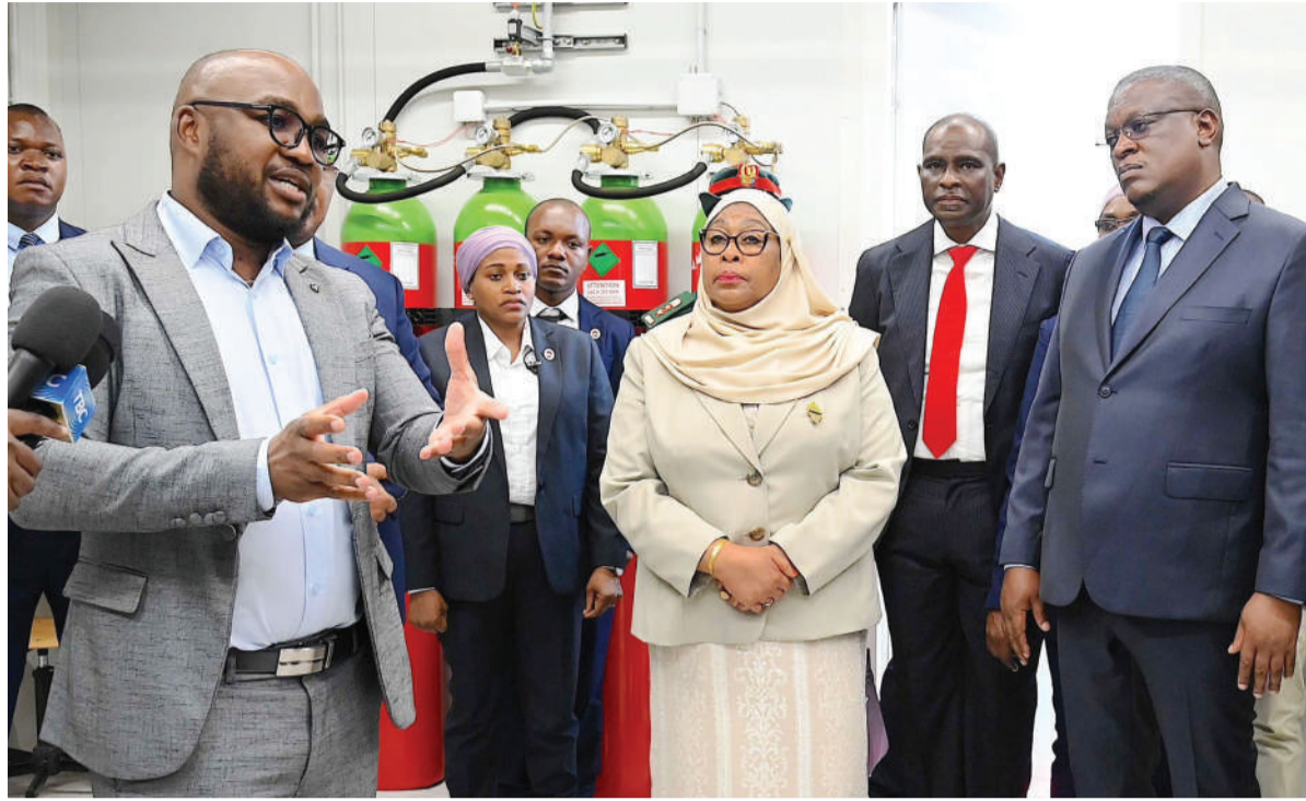
President Samia Suluhu Hassan gets explanation from Airtel Tanzania's chief technical officer Dr Prosper Mafale, at the launch of the Airtel 2Africa submarine cable station in Dar es Salaam on Thursday. Photo: Guardian Correspondent
