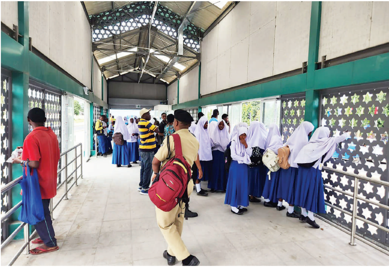
This is a scene at one of the modern stations built under Phase II of the Dar es Salaam Bus Rapid Transit project, covering the Gerezani-Sabasaba-Mtoni-Mbagala Kilwa Road stretch, as captured yesterday. Photo: Guardian Correspondent
