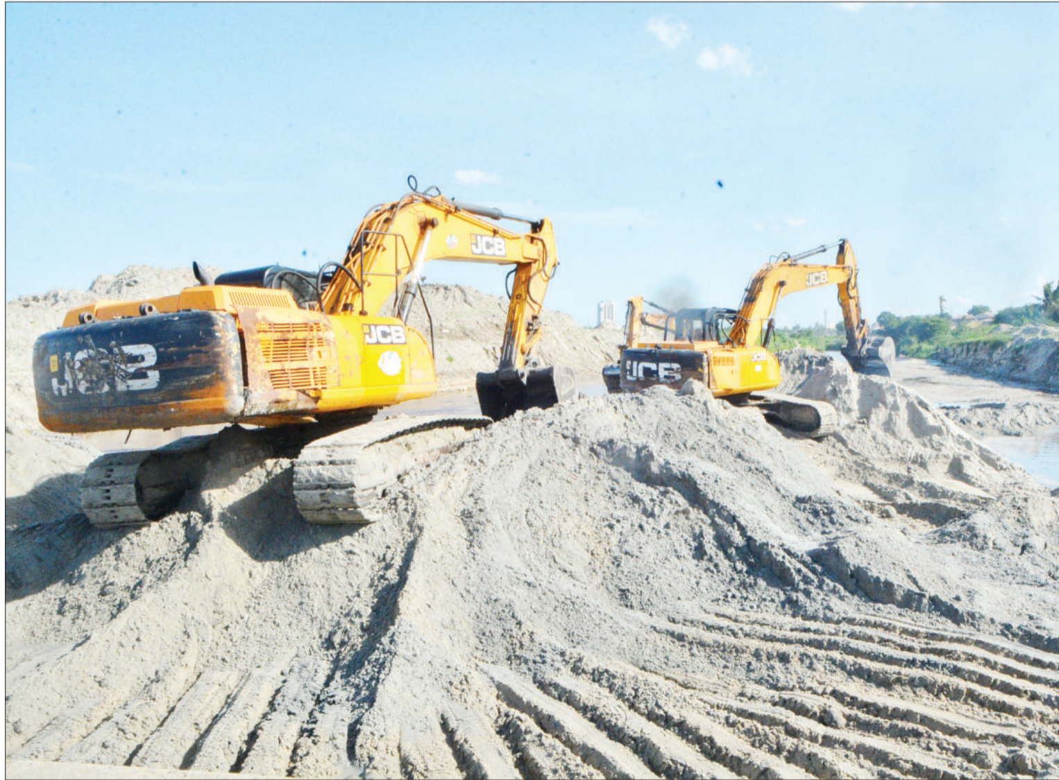
The Tanzania National Roads Agency (Tanroads) has begun scooping sand from clogged sections of Dar es Salaam's flood-prone Msimbazi and Jangwani valleys, with a view to easing the flow of water and effluent. Correspondent Miraji Msala captured the scene yesterday.
