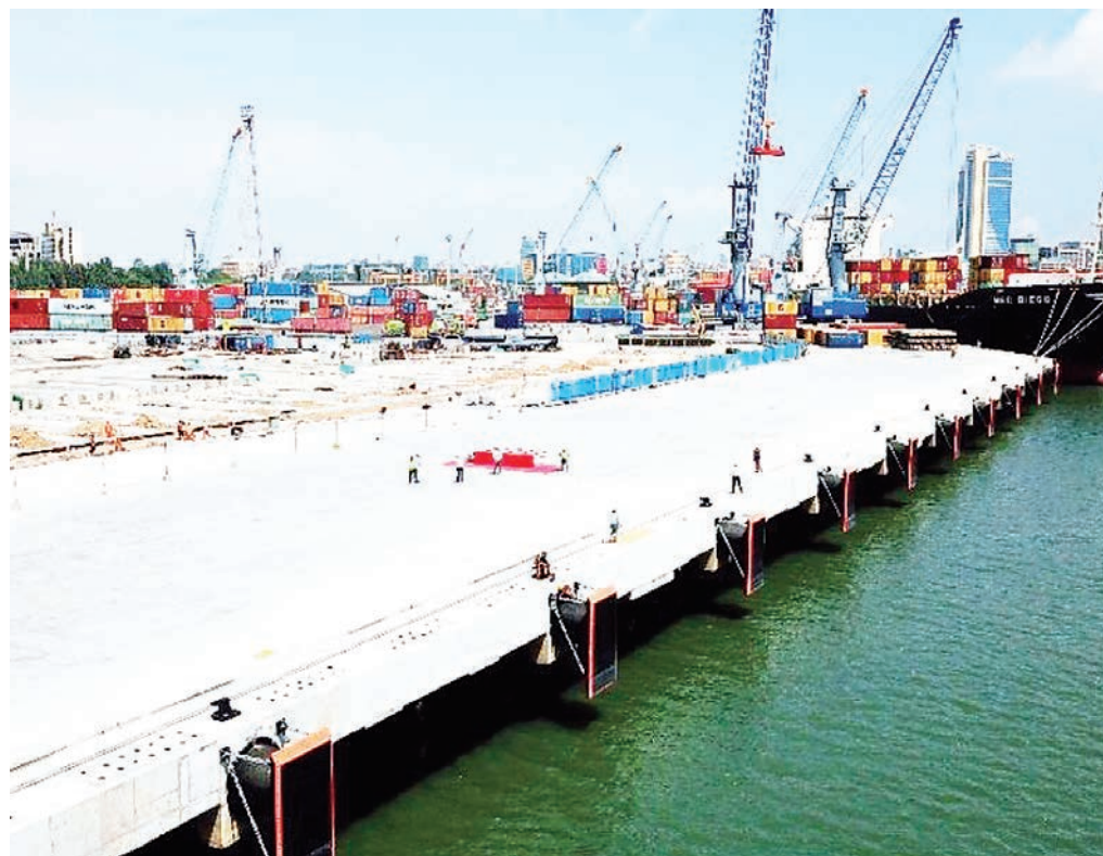
Newly constructed berth 5 at Dar port.
