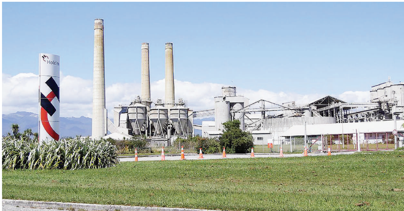
Holcim cement factory in Westport, New Zealand.
