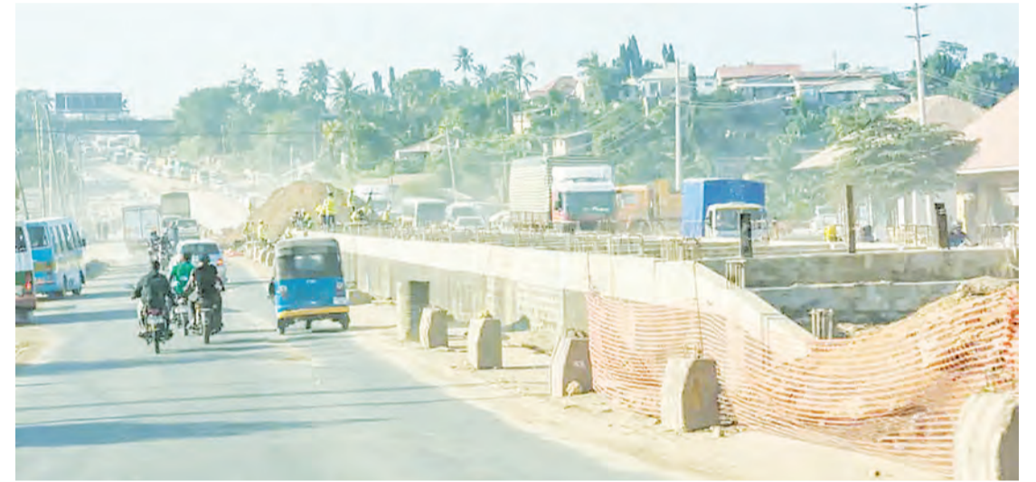
Ongoing constructions of BRT infrastructure in Dar es Salaam.
