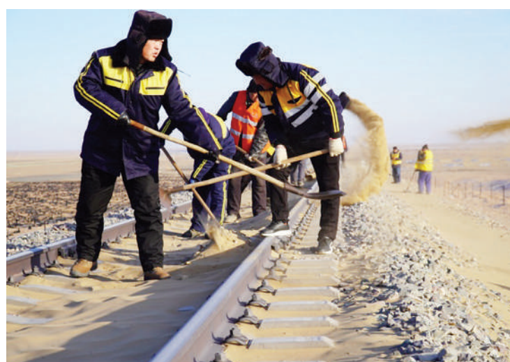
Desertification control staff clear sand off the tracks on the Linhai-Ceke railway in Alashan League, north China's Inner Mongolia Autonomous Region, Jan. 15, 2020. Tang Zhe/People's Daily
