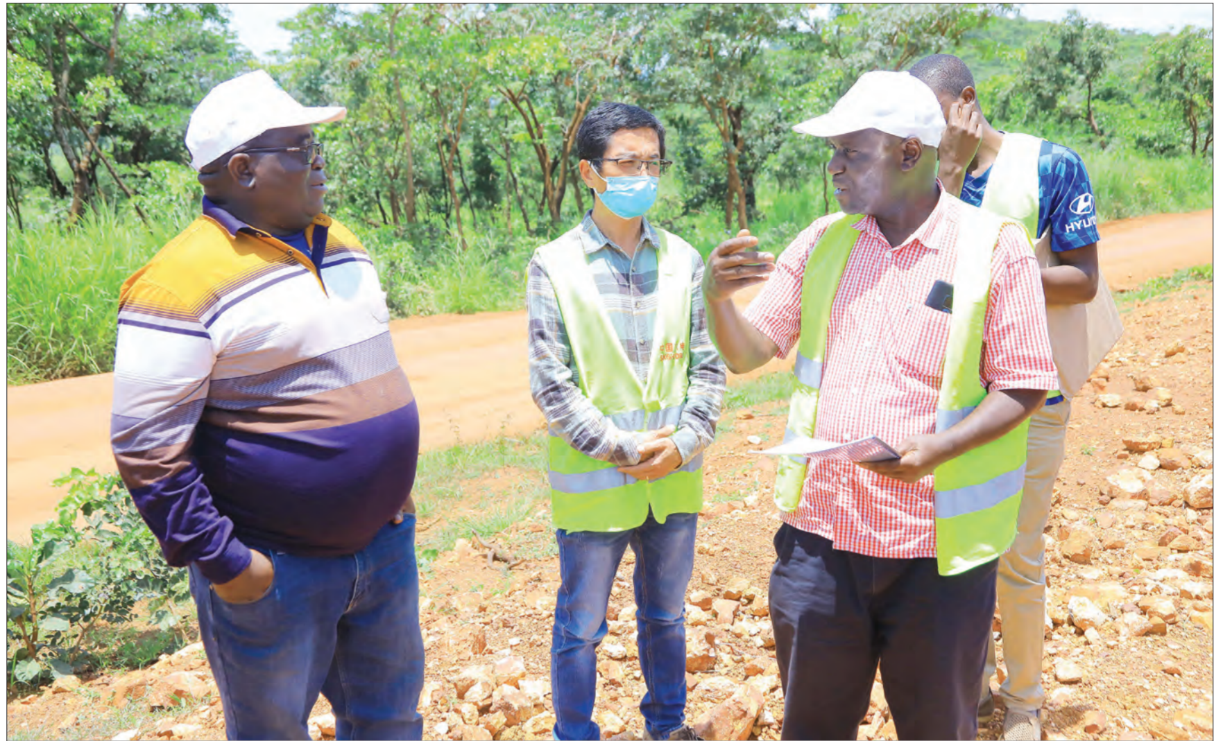
Feleki Amdi (gesturing), a consulting engineer with Kigoma Region's Nduta-Kabingo tarmac road project, makes an on-site briefing yesterday to Works and Transport deputy minister Godfrey Kasekenya (L) on the headway made in the work. Photo: Guardian Correspondent
