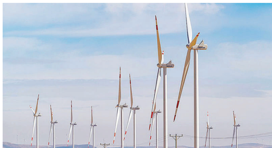
Wind turbines at a wind farm beside King's Highway in Ma'an Governorate in Jordan. Planned investment in Mena power sector slumped by a third amid the pandemic-driven slowdown this year.
