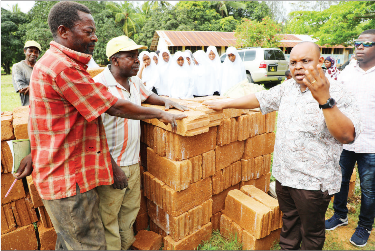
Uzini MP Khamis Hamza Chilo (R) hands over bricks for classrooms construction at Mchangani primary school yesterday. Photo: Guardian Correspondent
