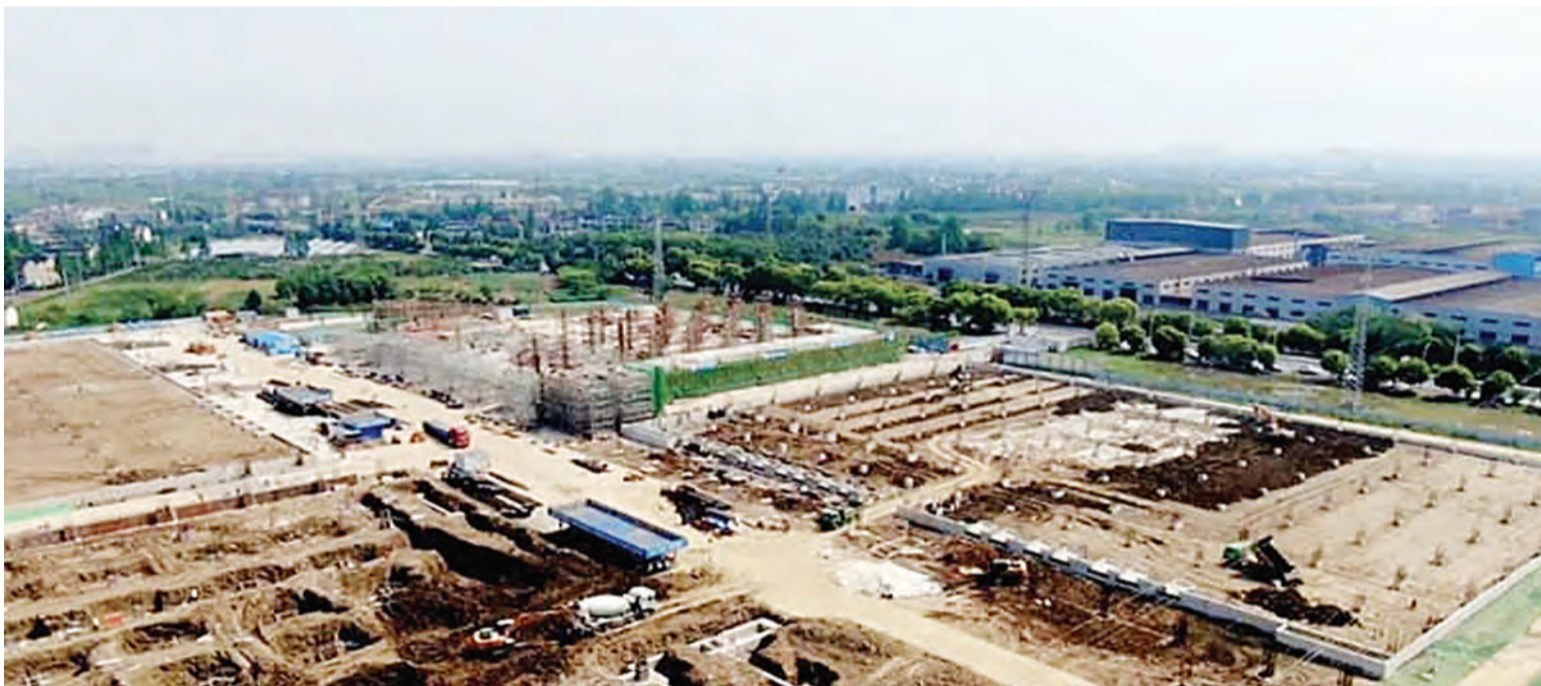
A Metcold facility in Changzhou, Jiangsu province under construction in 2020.
