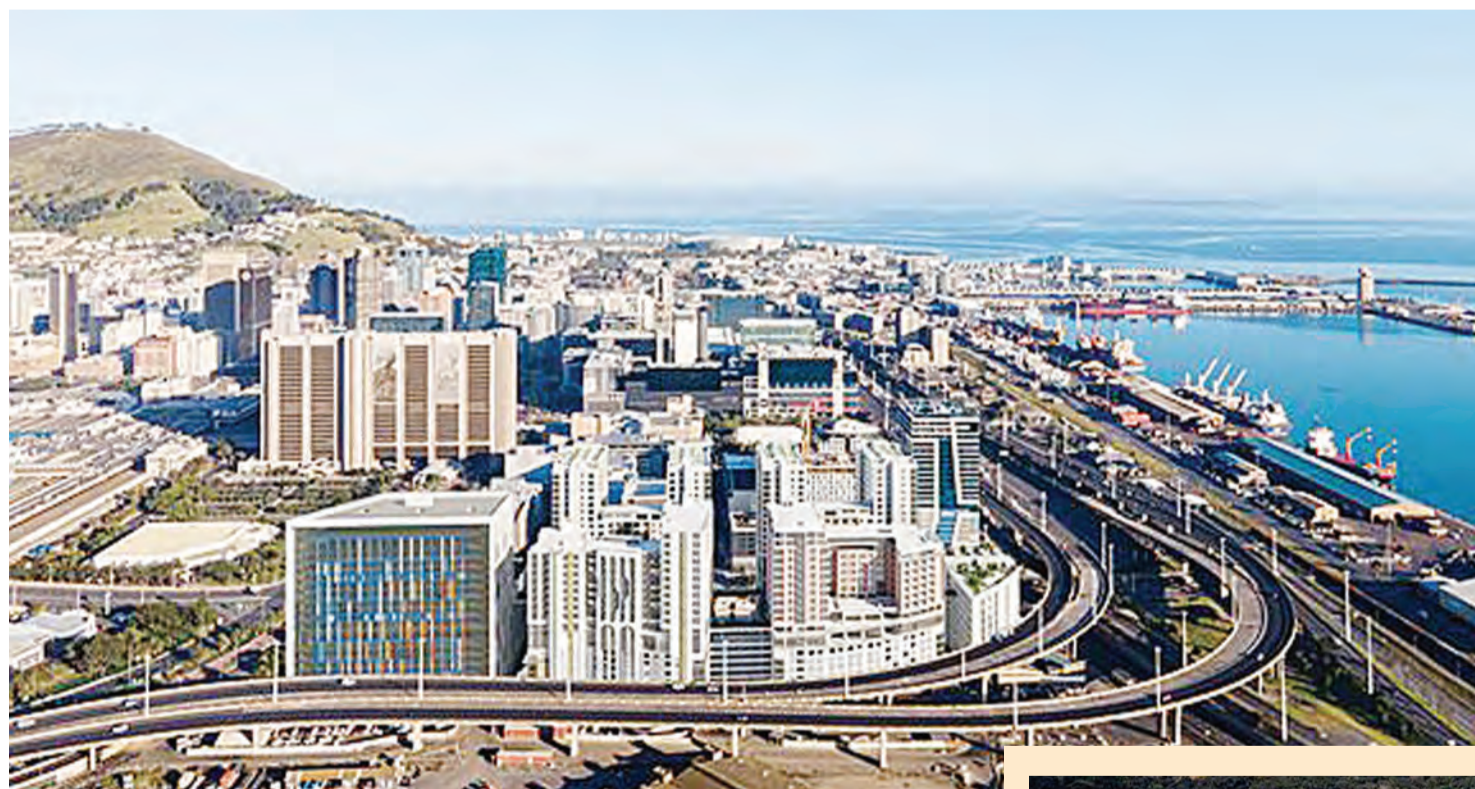
Harbour Arch taking shape on Cape Town's foreshore.
