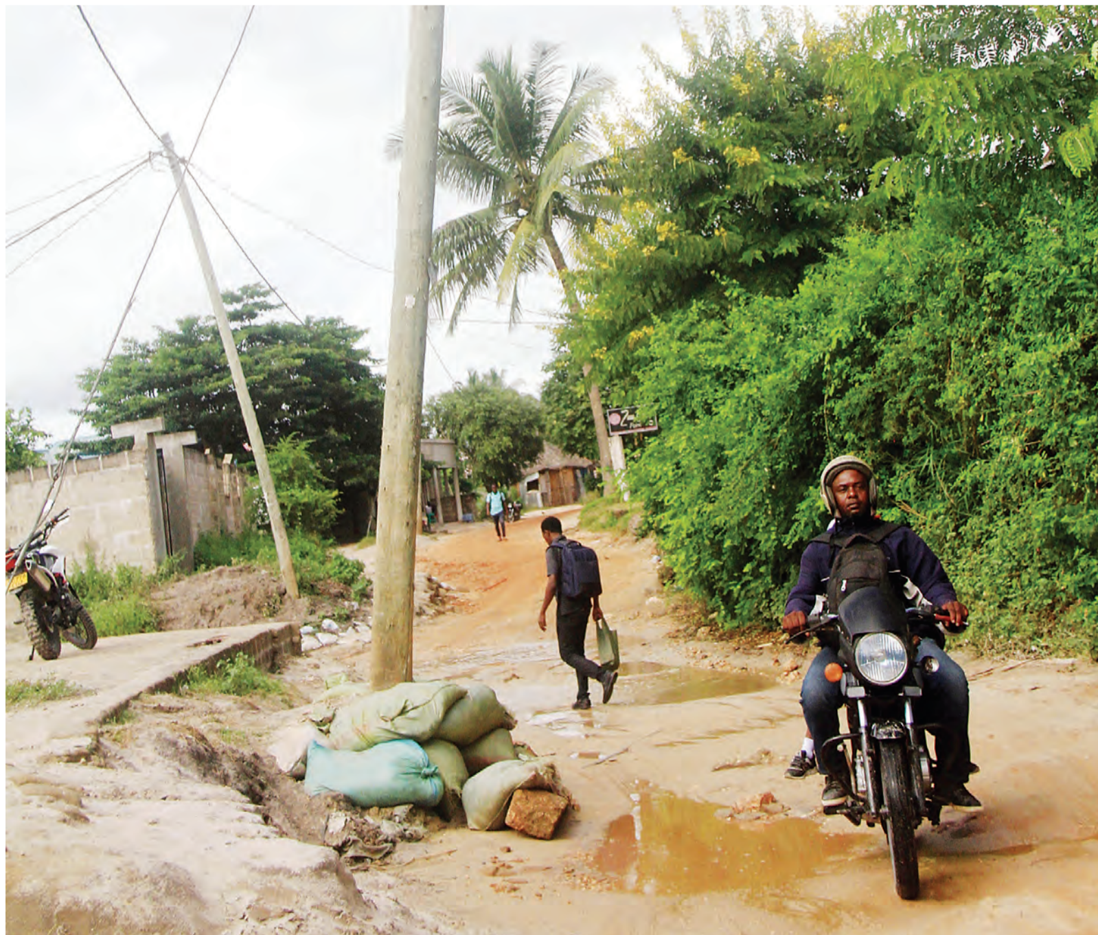
An unidentified volunteer places sandbags to hold an electricity transmission pole to prevent it from falling as it started to bend during ongoing rains at Kivule area on the southern outskirts of Dar es Salaam on Thursday. Photo: Correspondent Jumanne Juma
