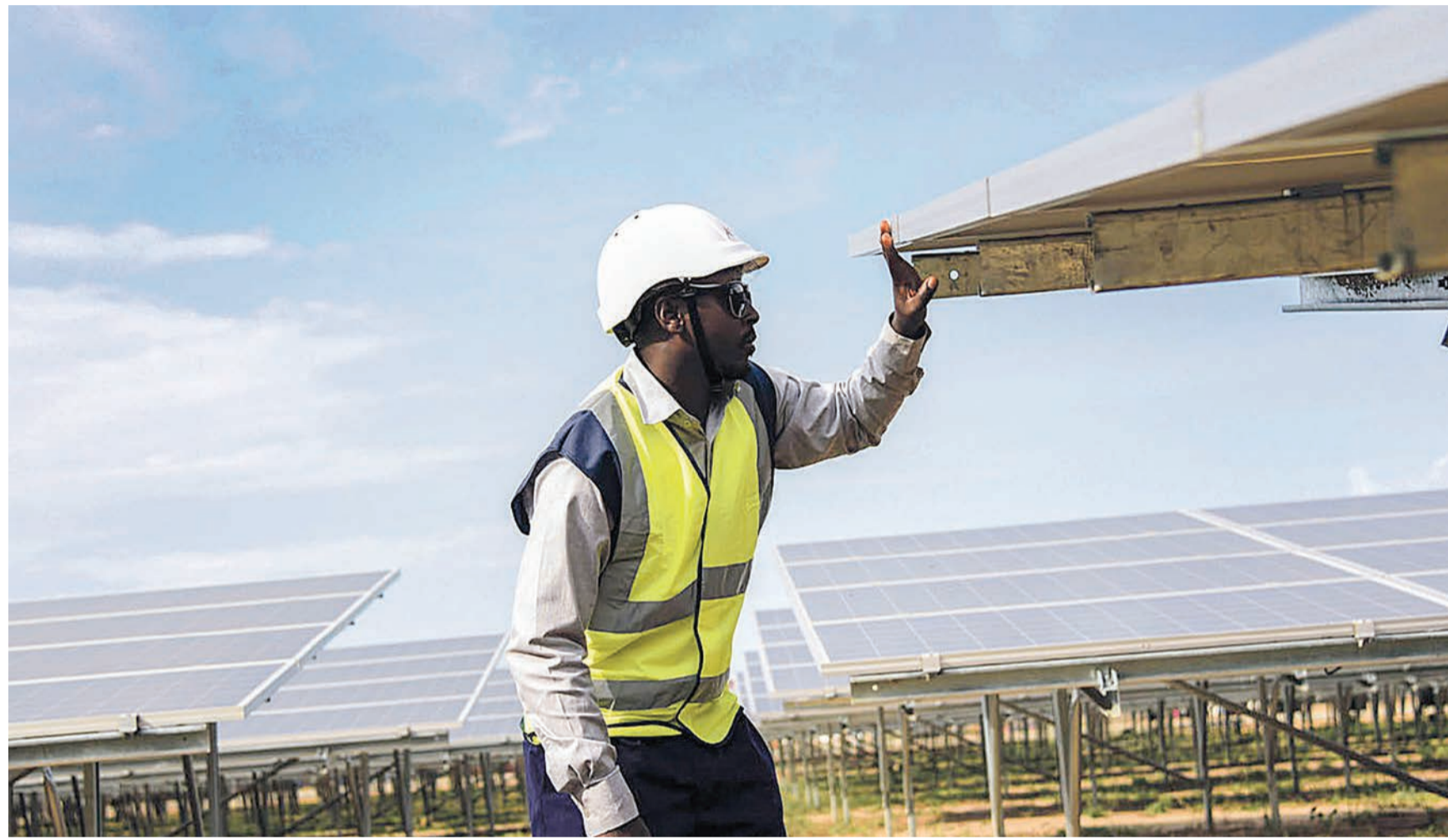
Access-Power's Soroti District solar plant with capacity of 50GW per annum is one of the largest in East Africa. File photo.
