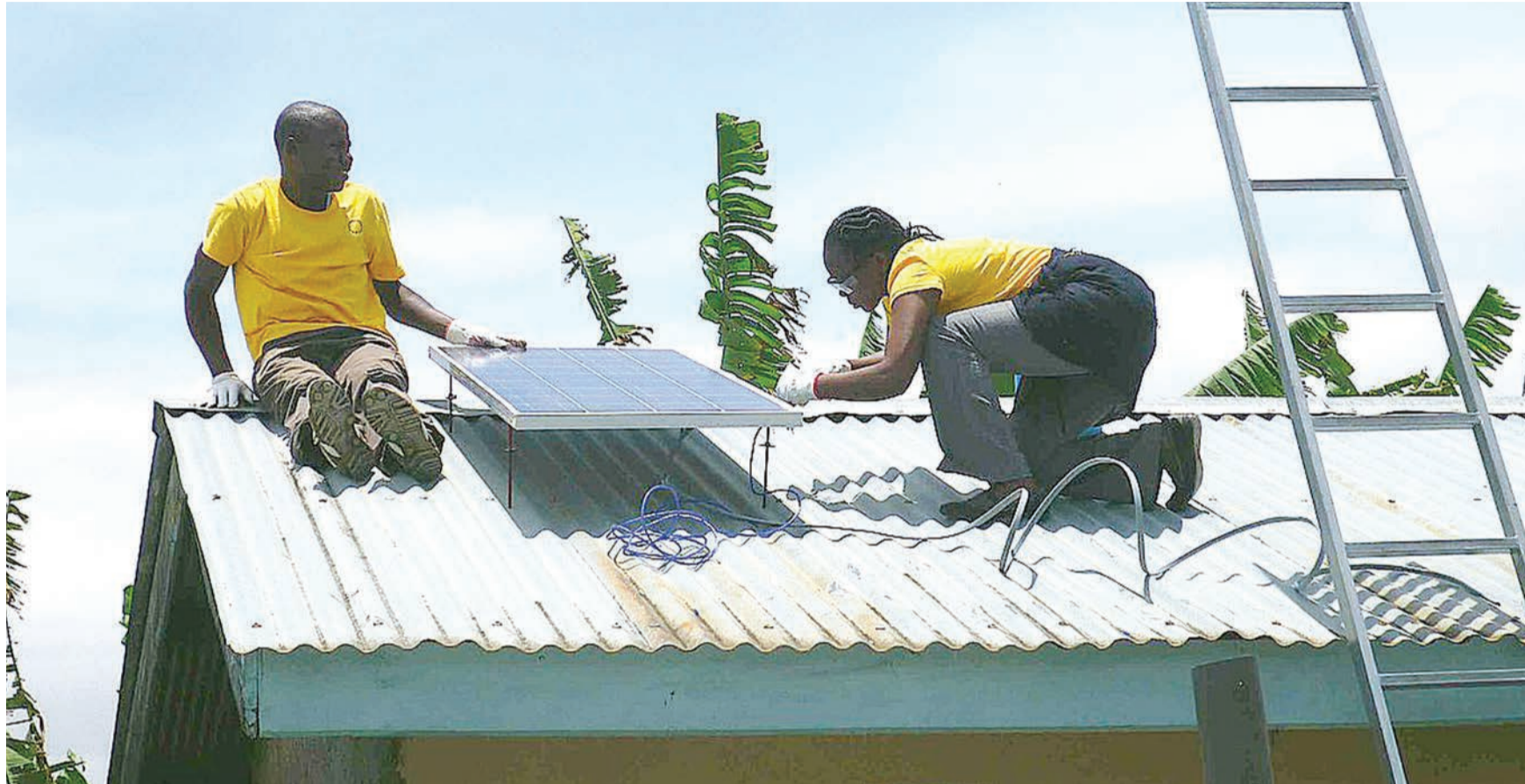
Mobisol Tanzanian technicians installing PV panel at a rural house in Arusha region.
