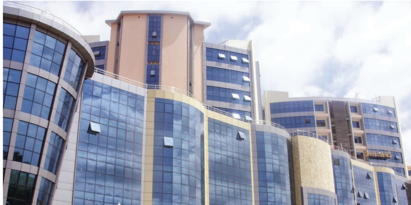
Kilimanjaro business complex
