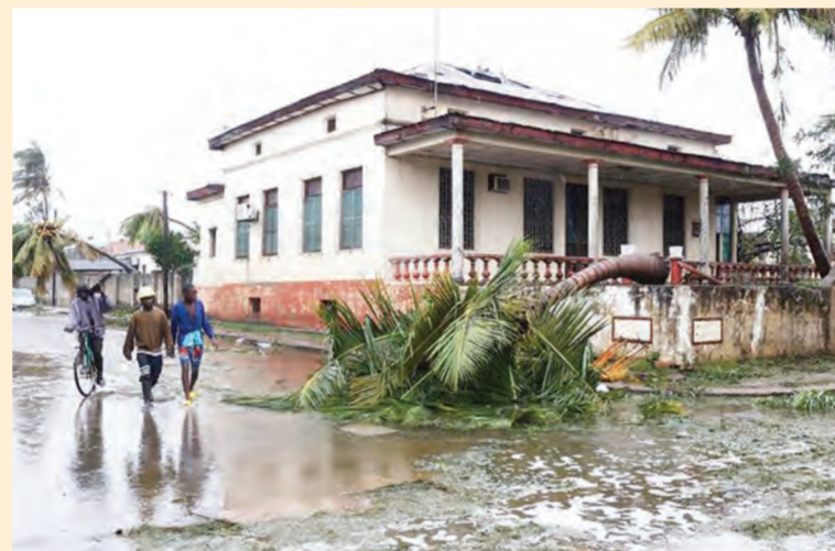
This handout photo taken and distributed by UNICEF on Sunday shows people walking along a street damaged by the impact of Cyclone Freddy in the city of Quelimane, Mozambique. AFP
