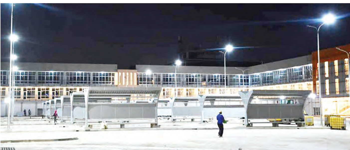
This is a view of a section of the modern complex mainly meant to serve as the new commuter bus stand at Mwenge in Dar es Salaam's Kinondoni municipality, as captured on Thursday night. It is understood that structure will also stand as a business hub. Authoritative sources said its construction is nearing completion, but they would not be drawn into saying precisely when it would become operational. Photo: Correspondent Miraji Msala
