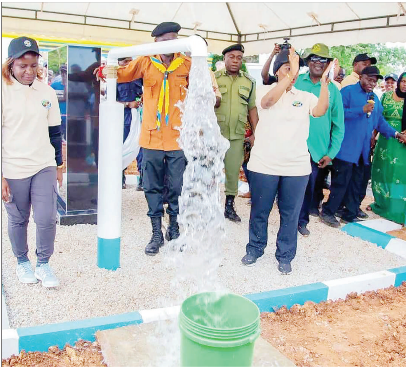
Uhuru Torch Race 2024 leader Godfrey Mnzava (C) turns on a tap in Tanga city's Chongoleani ward at the weekend to launch a water project implemented by Tanga Urban Water Supply and Sanitation Authority. Left is the agency's projects engineer, Violeth Kazumba, and right (applauding) is Health minister and Tanga Urban constituency legislator Umyy Mwalimu. Photo: Correspondent Oscar Assenga
