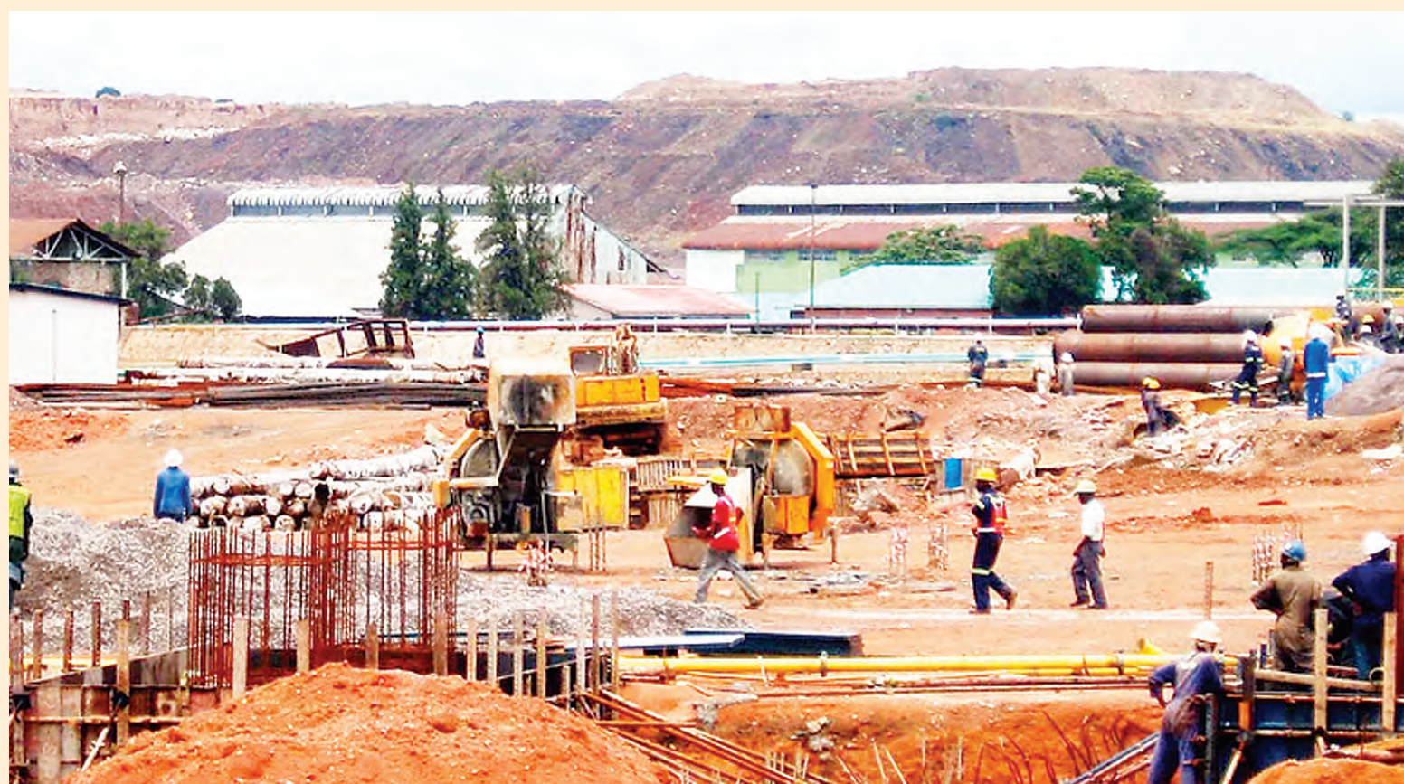
Workers build a copper foundry in Chingola, Zambia
