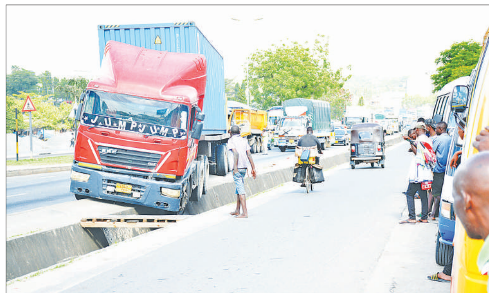
Traffic jam builds up along the EPZA stretch of Dar es Salaam's Mandela Road yesterday, with a heavy-duty truck having just about skidded off the road trying to steer clear of a gaping pothole. Photo: Correspondent Miraji Msala
