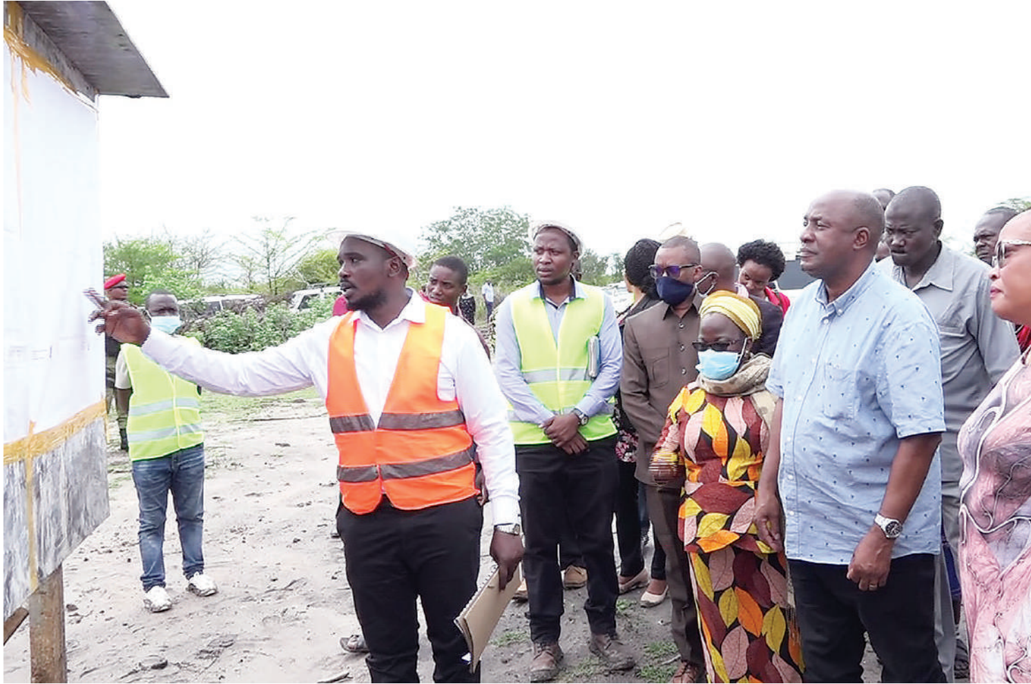
Livestock dip construction supervisor Robert Baltazar (L) shows Livestock and Fisheries deputy minister Pauline Gekul (R) on Wednesday the sketch of a dip lined up for Chamakweza at Chalinze in Coast Region, as Coast regional commissioner Evarist Ndikilo (2nd-R, foreground) looks on. Photo: Correspondent Mbaraka Kambona
