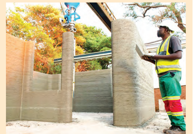
A 3D-printed house under construction
