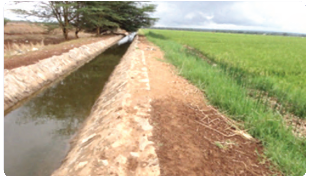
Completed repair work canal
