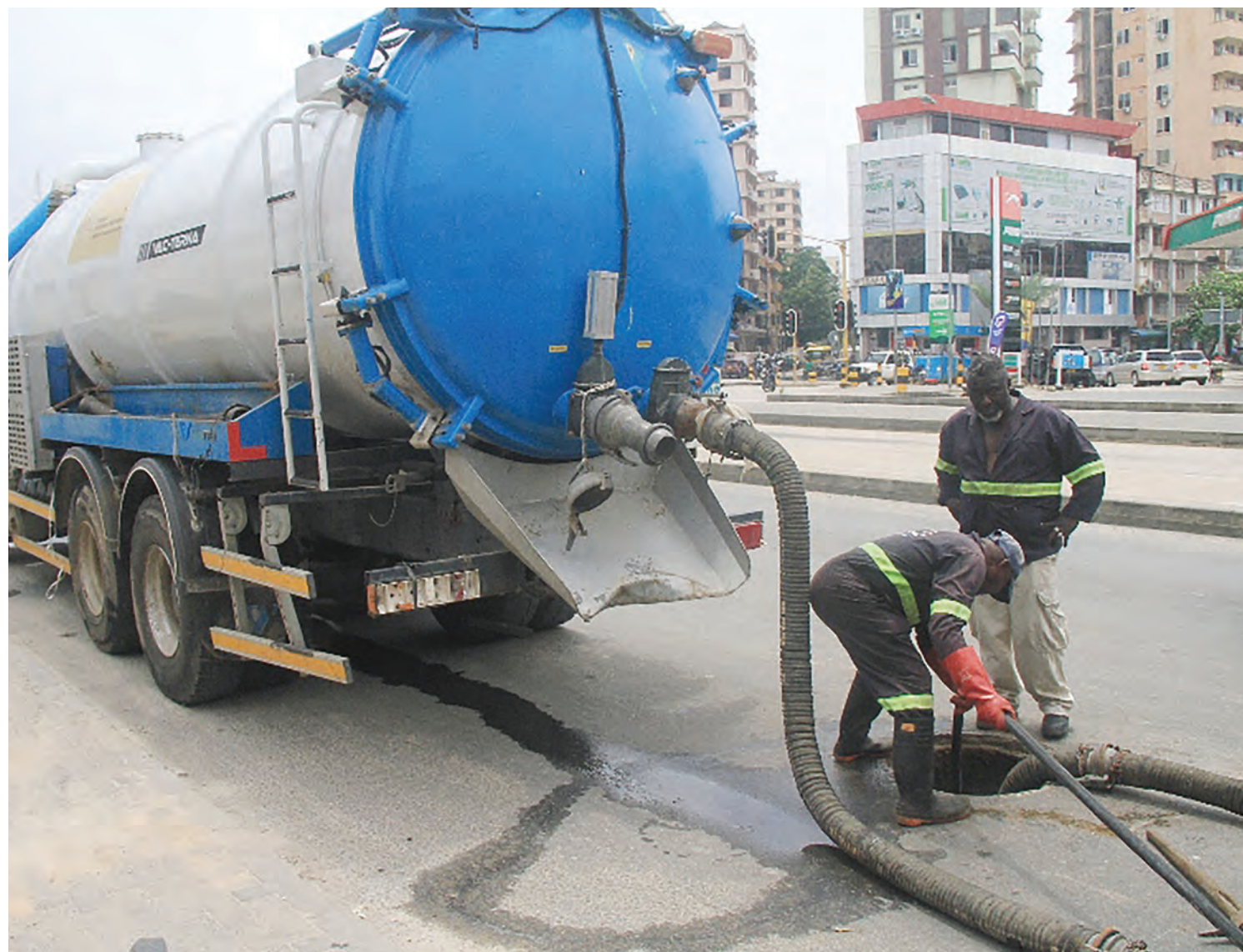
Dar es Salaam Water and Sewerage Authority (Dawasa) workers move to unclog a sewage system at a section of the city's Morogoro Road yesterday. Photo: Correspondent Jumanne Juma
