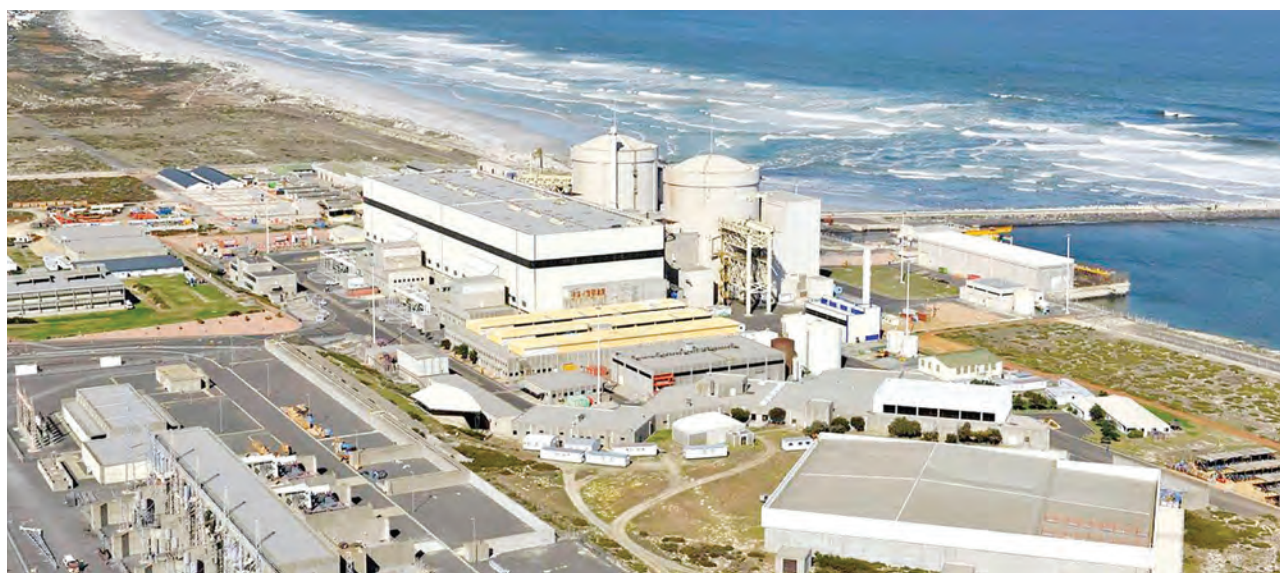
Koeberg nuclear power station. File Photo
