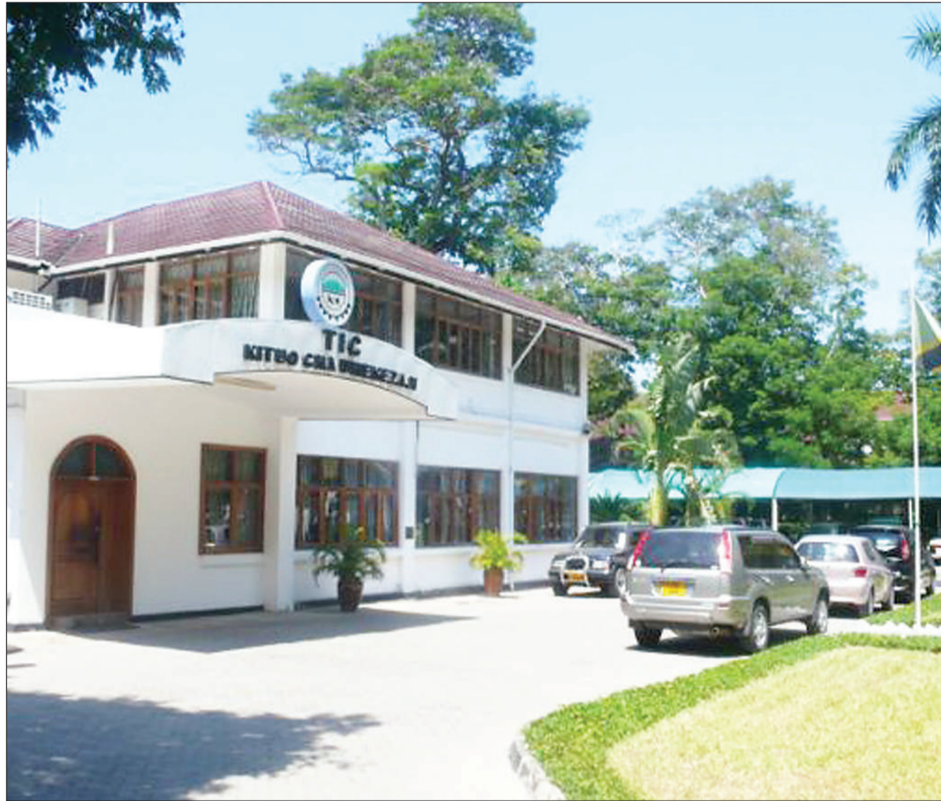
Tanzania Investment Centre headquarters in Dar es Salaam.
