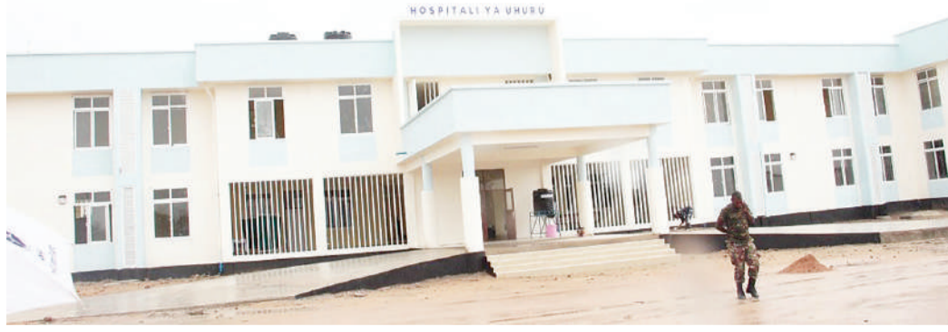
A newly built Uhuru Hospital in Chamwino District of Dodoma Region.
