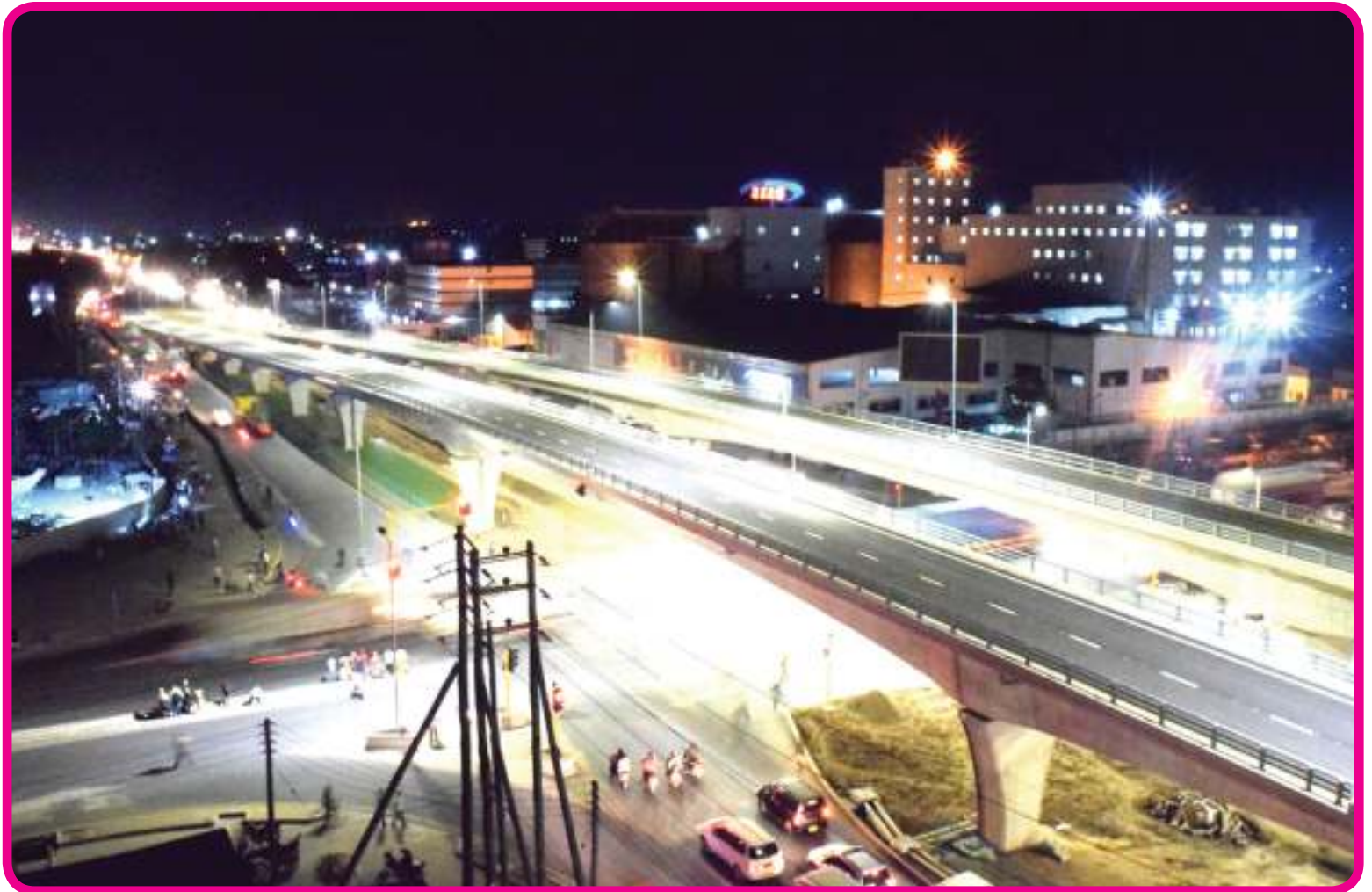
Night scene of Mfugale flyover
