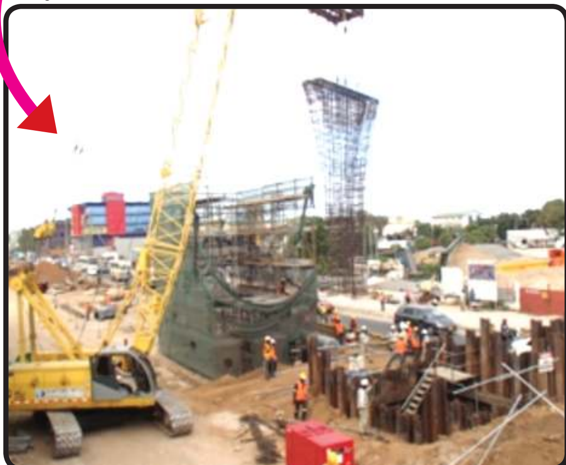
Construction was done collaboratively by Tanzanian workers and Japanese contractor.
