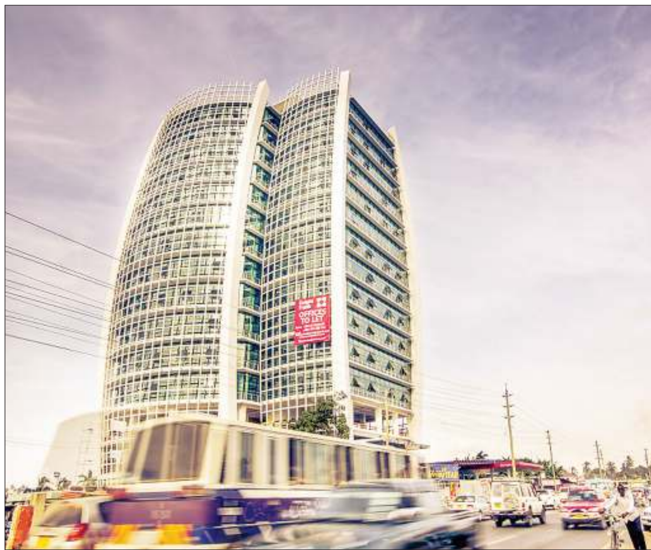
The TanHouse commercial building in Dar es Salaam remains largely vacant.
