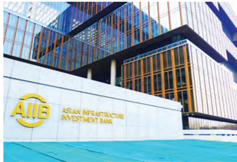
Asian Infrastructure Investment Bank headquarters in Beijing
