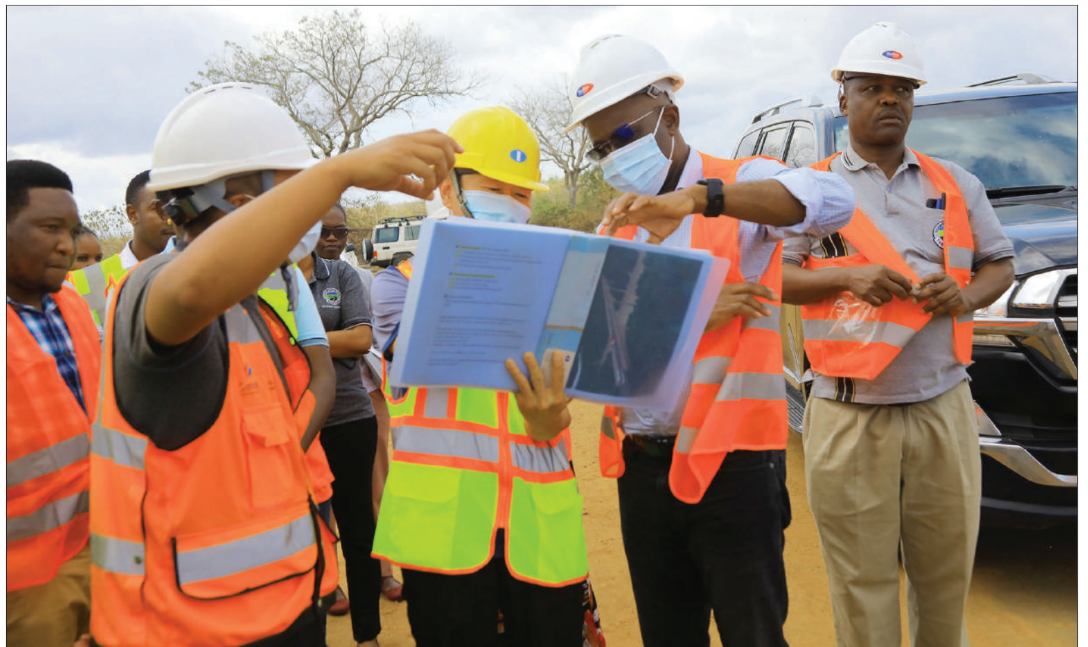
Works and Transport minister Prof Makame Mbarawa (L) pictured yesterday at the site of Wami Bridge in Coast Region flipping through work plan documents on the strategic structure - which is undergoing major works. Photo: Guardian Correspondent
