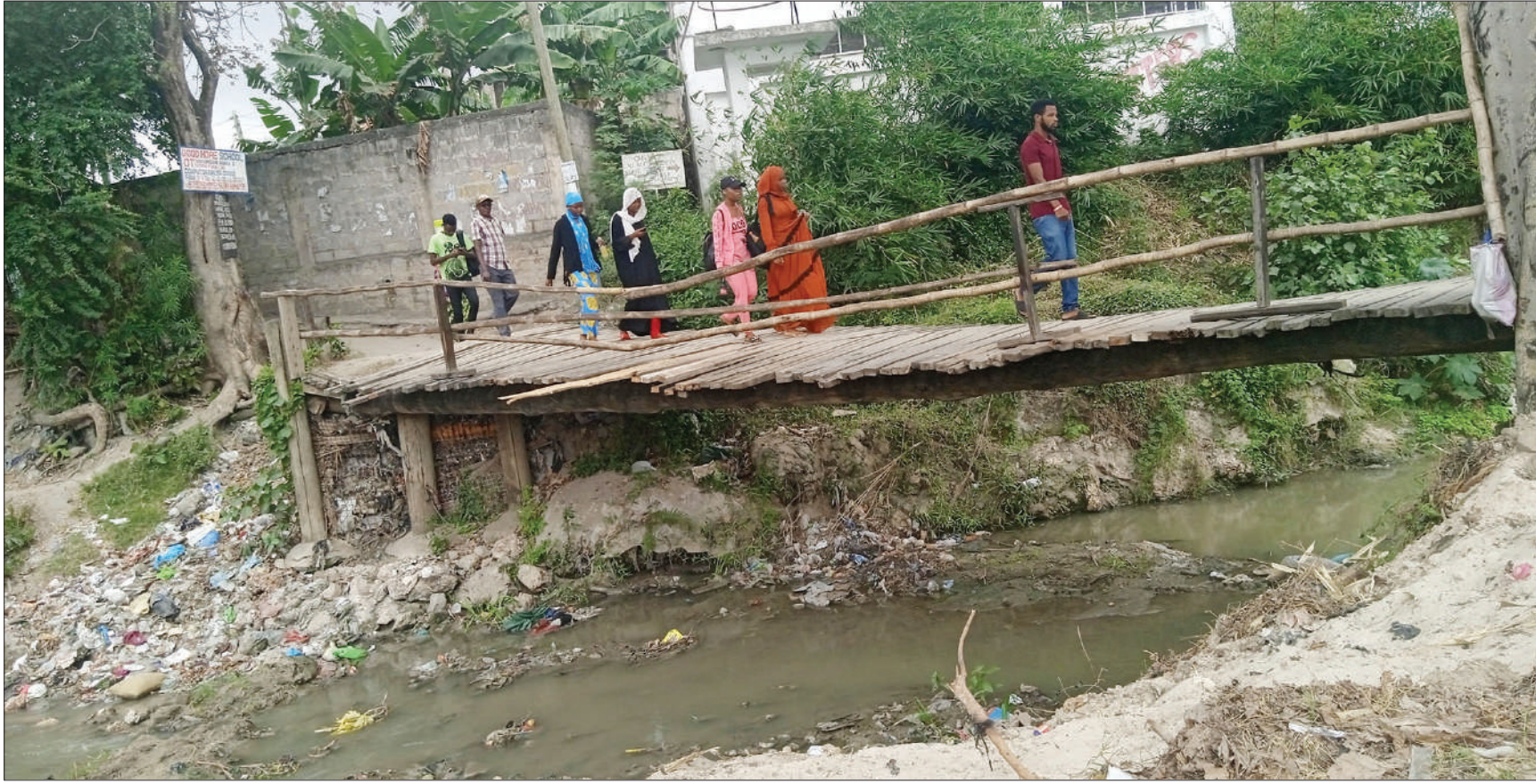
With a better option nowhere around, these residents of Bondeni in Dar es Salaam's Ubungo ward make do with this makeshift bridge connecting Ubungo National Housing and Sinza Mawasiliano. Sources say it was assembled by one Azizi Madaraji. Photo: Owen Bariki of TUDARCO
