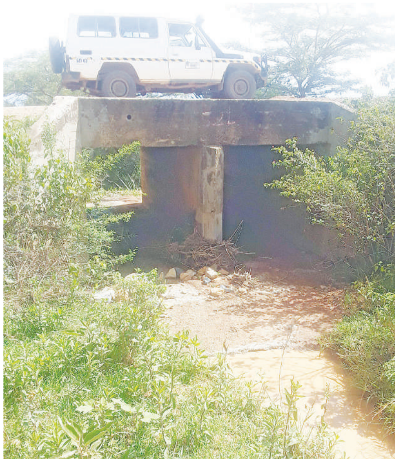
Gokohe River Bridge
