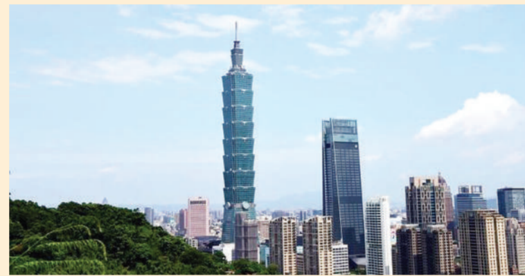
This undated file photo shows the Taipei 101 skyscraper in Taipei. (PHOTO / XINHUA)
