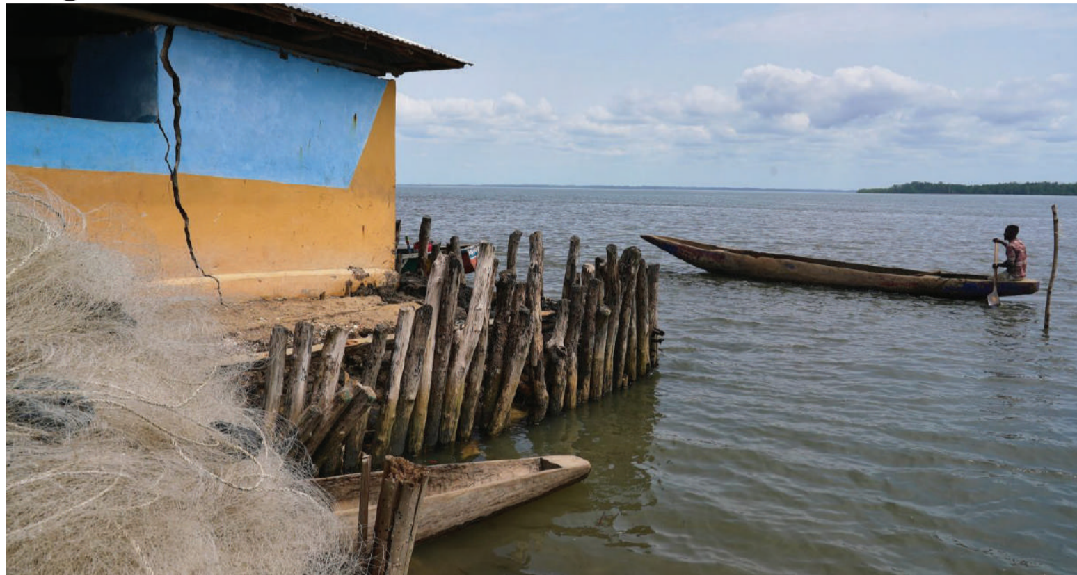
A makeshift seawall built with mangrove wood in Sherbro estuary.
