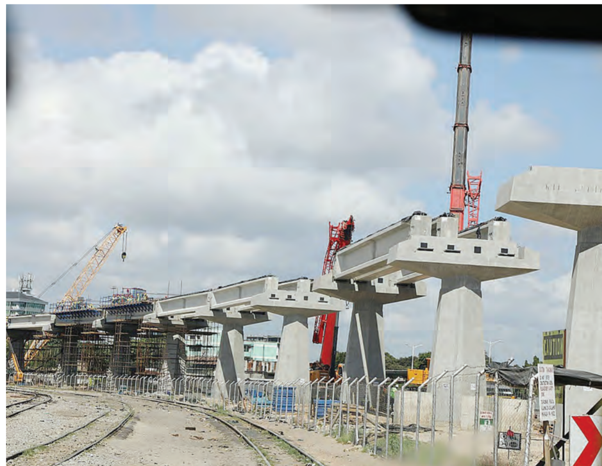
Ongoing construction of SGR infrastructure
