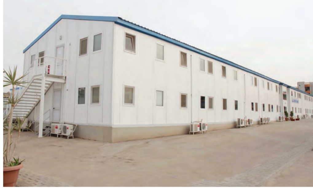
Prefabricated building in Tanzania
