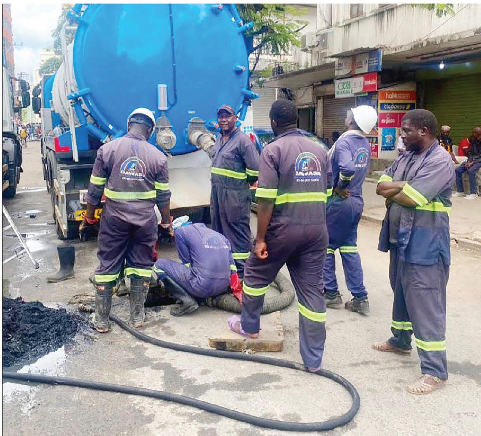
Dar es Salaam Water and Sanitation Authority (Dawasa) technicians unclog a sewage system in the city yesterday. Photo: Correspondent Joseph Mwendaipole
