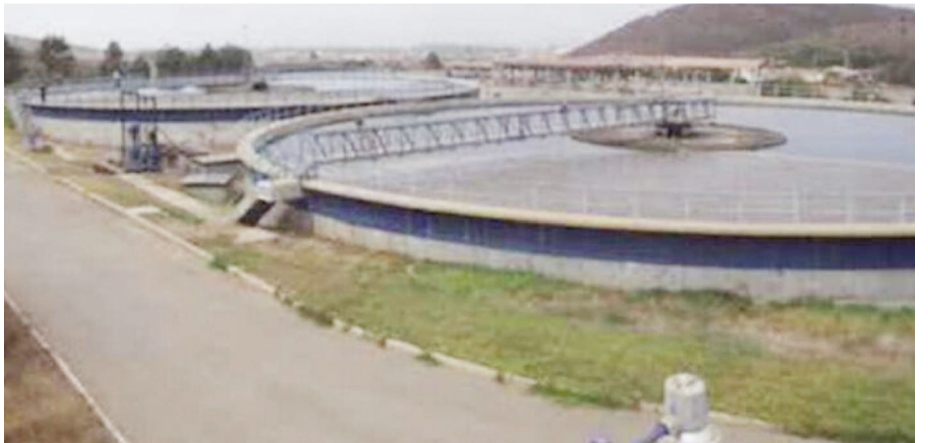
The El Naranjo municipal treatment plant in the city of Ensenada, in the northwestern peninsular state of Baja California, is operating below its installed capacity, which is further affecting the distribution of scarce water in the city. CREDIT: Conagua
