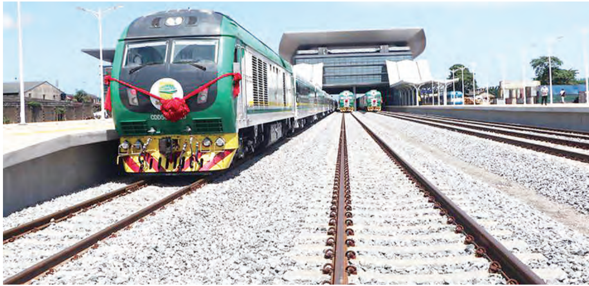
Trains park on the track at the Mobolaji Johnson Railway Station of the Lagos-Ibadan railway in Lagos, Nigeria, on June 10, 2021. China-Africa cooperation is bearing fruits and unleashing huge potential with the high-quality implementation of the “eight major initiatives.” Put forward at the Beijing summit of the Forum on China-Africa Cooperation (FOCAC) held in September 2018, the eight major initiatives cover the fields of industrial promotion, infrastructure connectivity, trade facilitation, green development, capacity building, health care, people-to-people exchanges as well as peace and security. Xinhua
